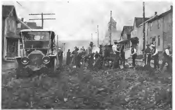
Road Makers Preparing the Way at Johnstown.
